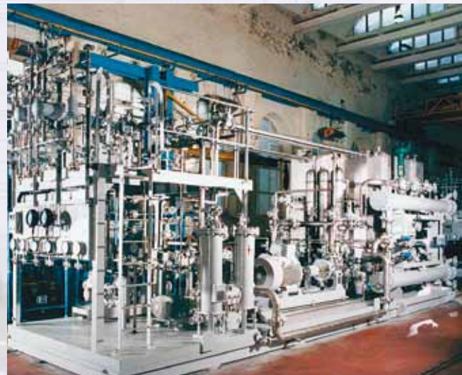
Compressed air cooling
