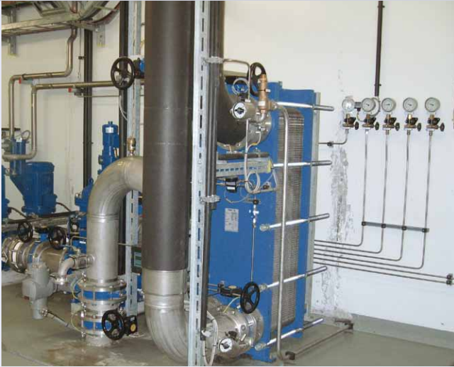
Hydraulic oil cooling in power plant.
