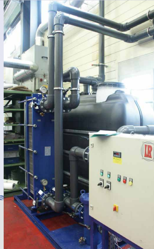
Cooling of lubricating oil for extruding presses.
